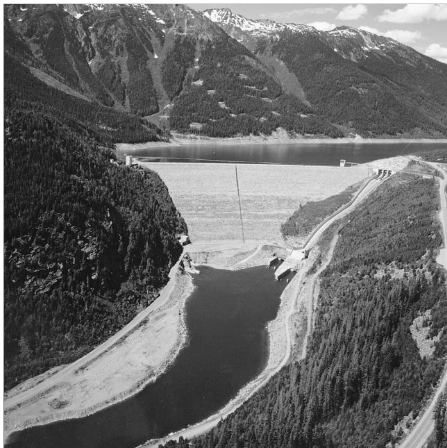
Mica Dam in British Columbia was built to provide 7 million acre feet of water storage as outlined in the Columbia River Treaty, plus another 5 million acre feet referred to as “non-treaty storage.” In comparison, Grand Coulee Dam in Washington has 5.2 million acre feet of storage.
